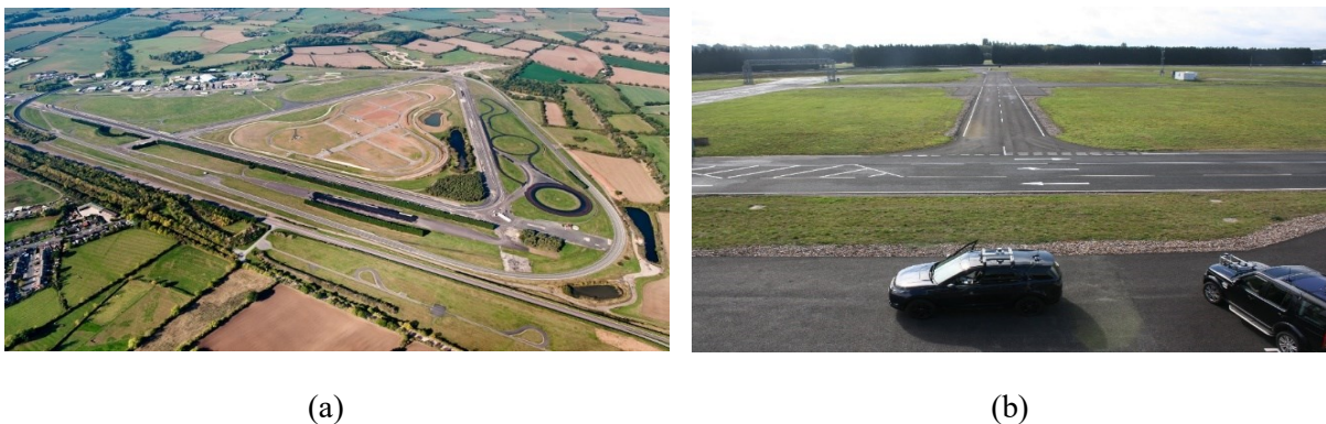
Figure 1: Pictorial representation of the test area. (a) Google Map plan view. (b) Panoramic photo.
